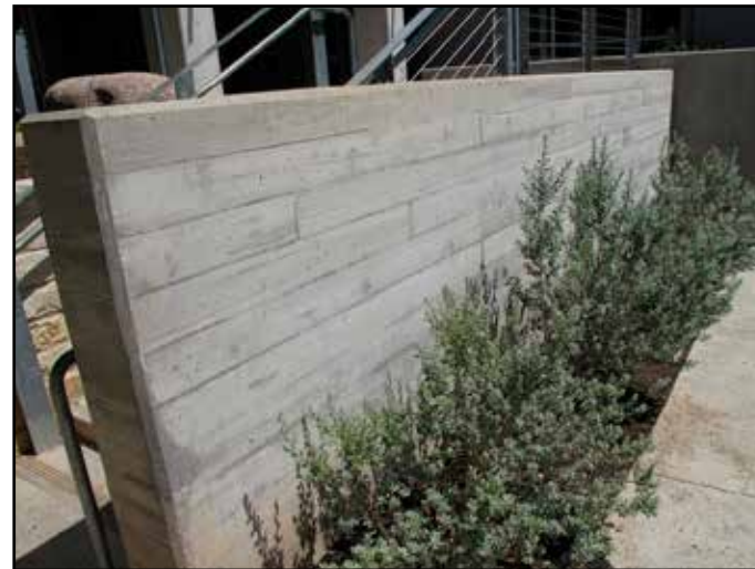
Retaining Wall Veneer
